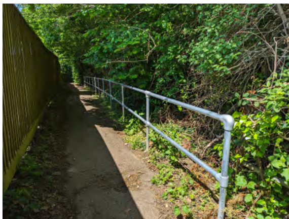
New safety railings along Dince Hill Close footpath
